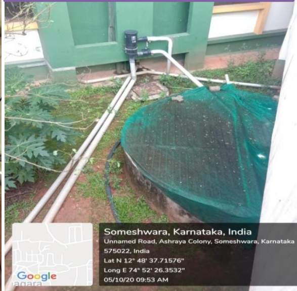
Open Well In front of Gardyenia B block
